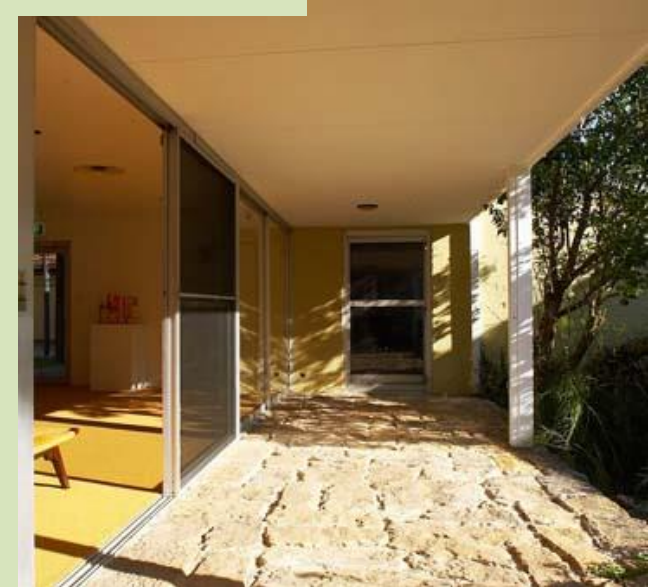
Side view of Ancher House
